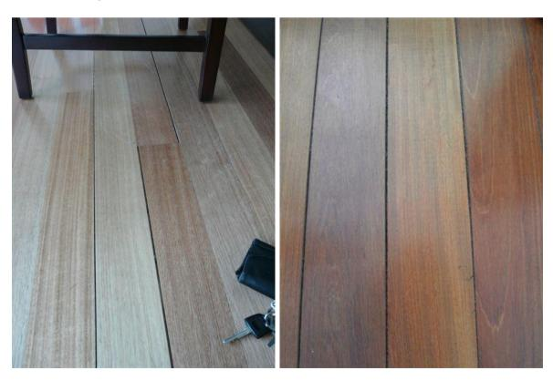
And in the latter scenario as the rainy season is in full swing and the floor boards absorb the air moisture and grow wider in size the floor may soon become too wide for the room in which it is installed and then get forced
