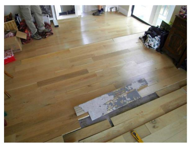
The above two scenarios are a direct cause of humidity failure. The shrinkage situation may be considered somewhat normal for solid wooden flooring and will close up again in the wet season but the bursting of the floors in the latter situation will need an expensive repair and in some cases a full replacement.
